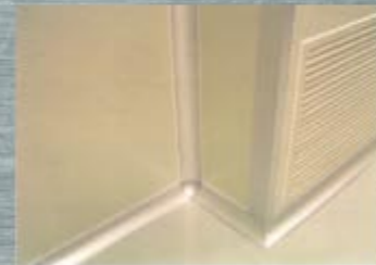
COVING FINISHES FOR FLOOR, WALL AND CEILING
